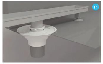
**Step 11.** Place the drain base into the threaded nipple. Use the adjustable feet to keep the drain channel into the correct position and level.
