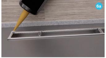
**6a.** Once grate and slider position are verified, apply sealant around the top edge of the base and thin-set to the bottom of the grate, or remove the paper backing from the sealant tape.
