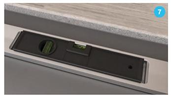
**Step 7.** Verify that the grate is perfectly straight and level before installing the floor. Use enclosed wedges to raise any part of the grate if needed.
